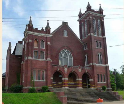
Note: This is the front entrance of the now-dilapidated church (Elmalvaney, 2011).
